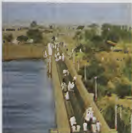
The Sannār Dam on the Blue Nile River in the Sudan
